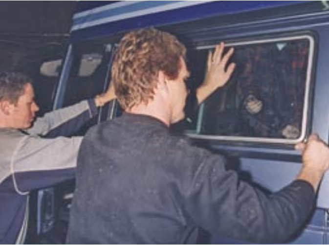
2-2-27. They're there for a very important reason: the glass has to be pushed firmly inwards as the rubber lip is pulled over the panel on the inside.
