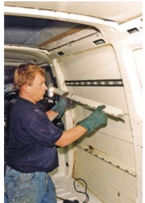
2-2-4. Barry now removes the rail exposing the panel to be cut away.
